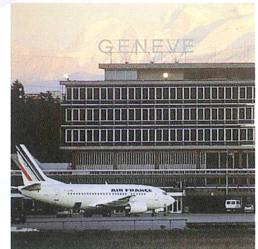
Geneva Airport FAFCO Ice Bank Storage capacity: 17 700 kWh
