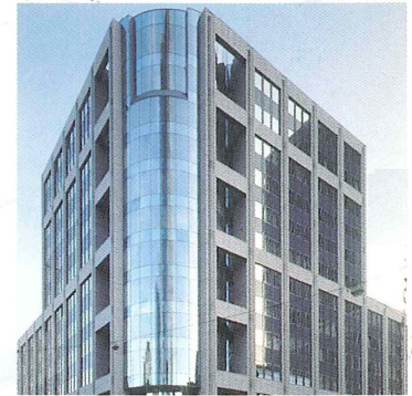
Bayrische Vereinsbank, Frankfurt FAFCO Ice Bank Storage capacity: 8000 kWh
